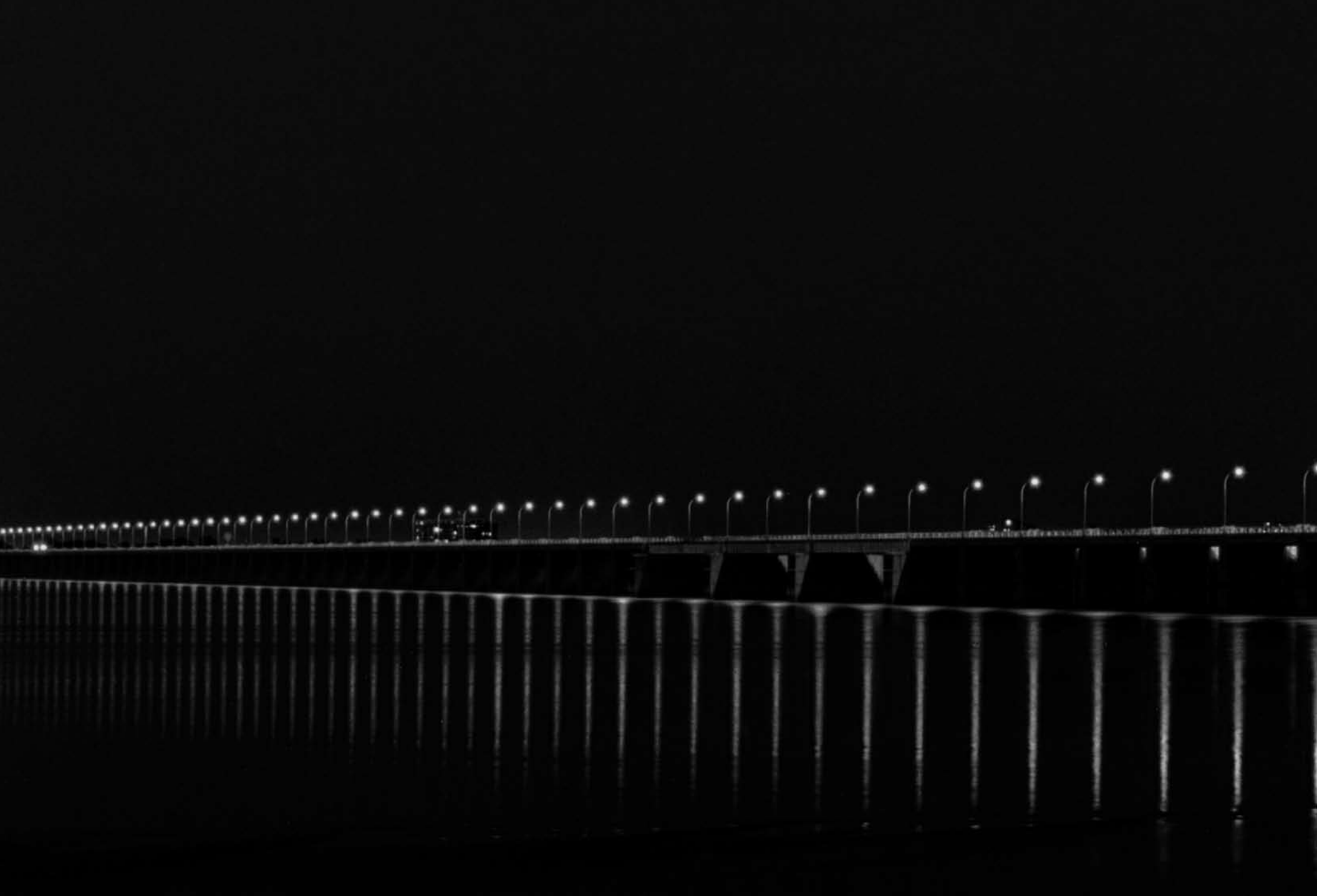
Champlain Bridge Ice Breaking Structure (Estacade) in Montreal.
