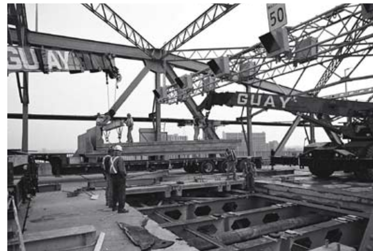
↑ The Jacques Cartier Bridge deck replacement that took place in 2001-2002 will serve as a model for the Honoré-Mercier Bridge rehabilitation.
