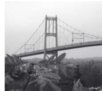
↑ The Thousand Islands International Bridge
