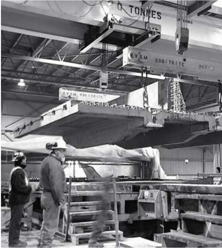
↑ The use of prefabricated deck panels, which proved efficient during the deck replacement of the Jacques Cartier Bridge, will also be used for the rehabilitation of the Honoré Mercier Bridge.
