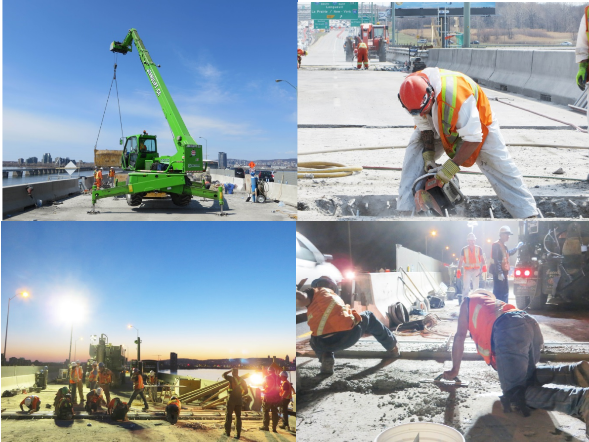
Joint replacement project at the Champlain Bridge in Montreal
