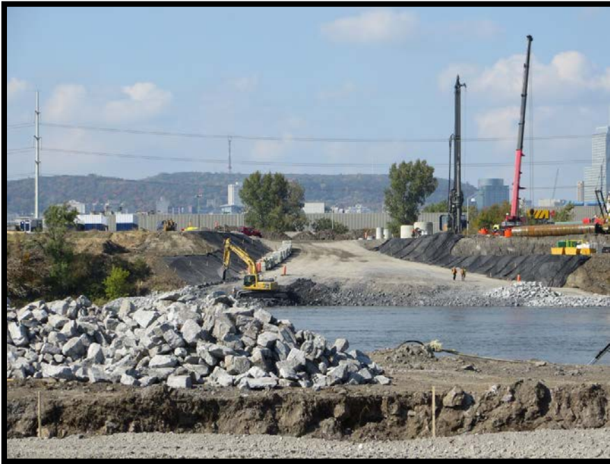
At the top, model of the new île des Sœurs temporary bridge in Montreal, and beginning of the construction of the access.
