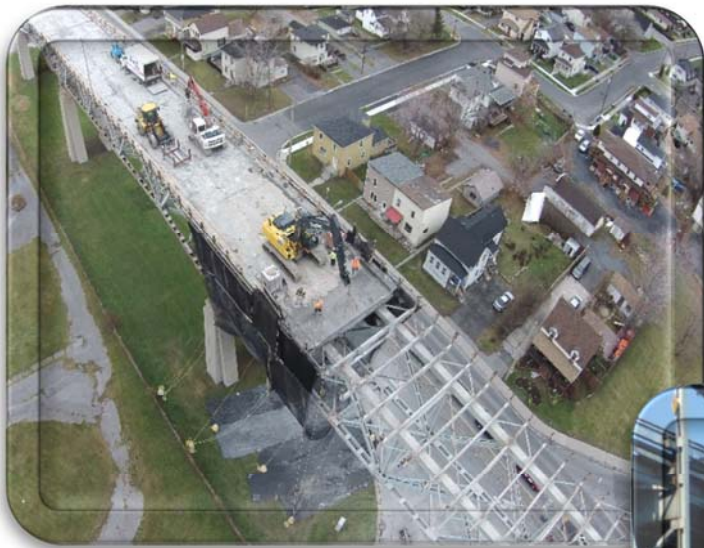
Concrete deck removal at the North Channel Bridge in Cornwall in late November.
