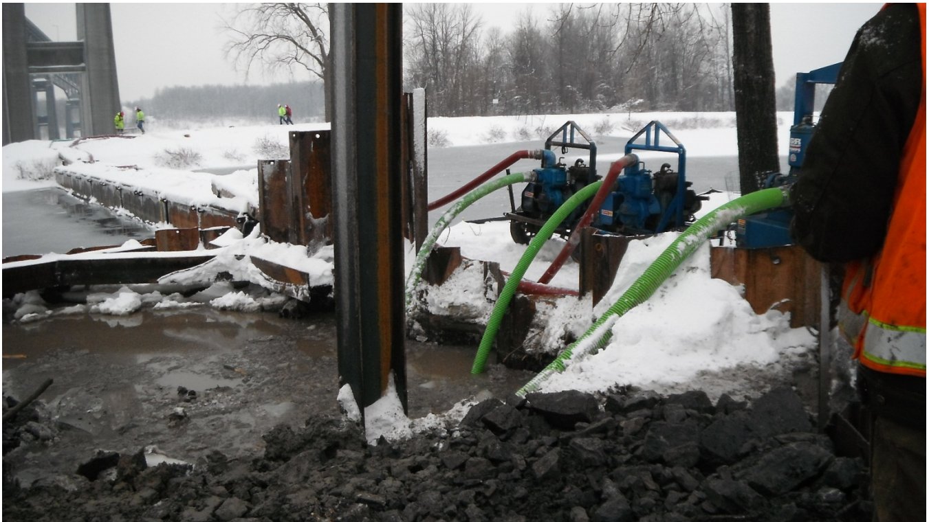
Pumping out water from inside the cofferdam (north abutment of the new North Cannel Bridge in Cornwall).
