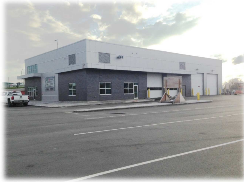
Completed Maintenance Building in Sault Ste. Marie, Ontario
