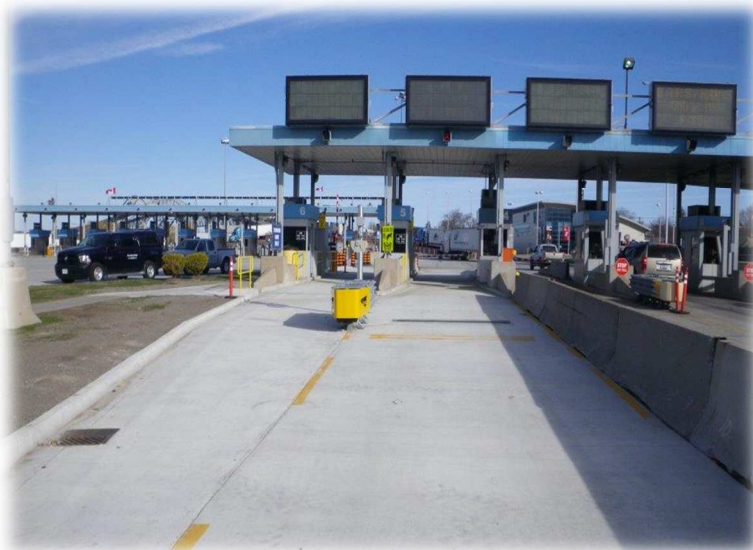
View of the completed Deck Resurfacing Project and the new and ongoing automated toll lanes at the Blue Water Bridge in Point Edward
