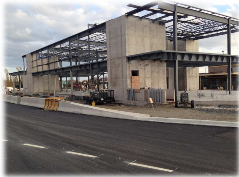
Construction (steel erection) of the CBSA Traffic Building in Sault Ste. Marie
