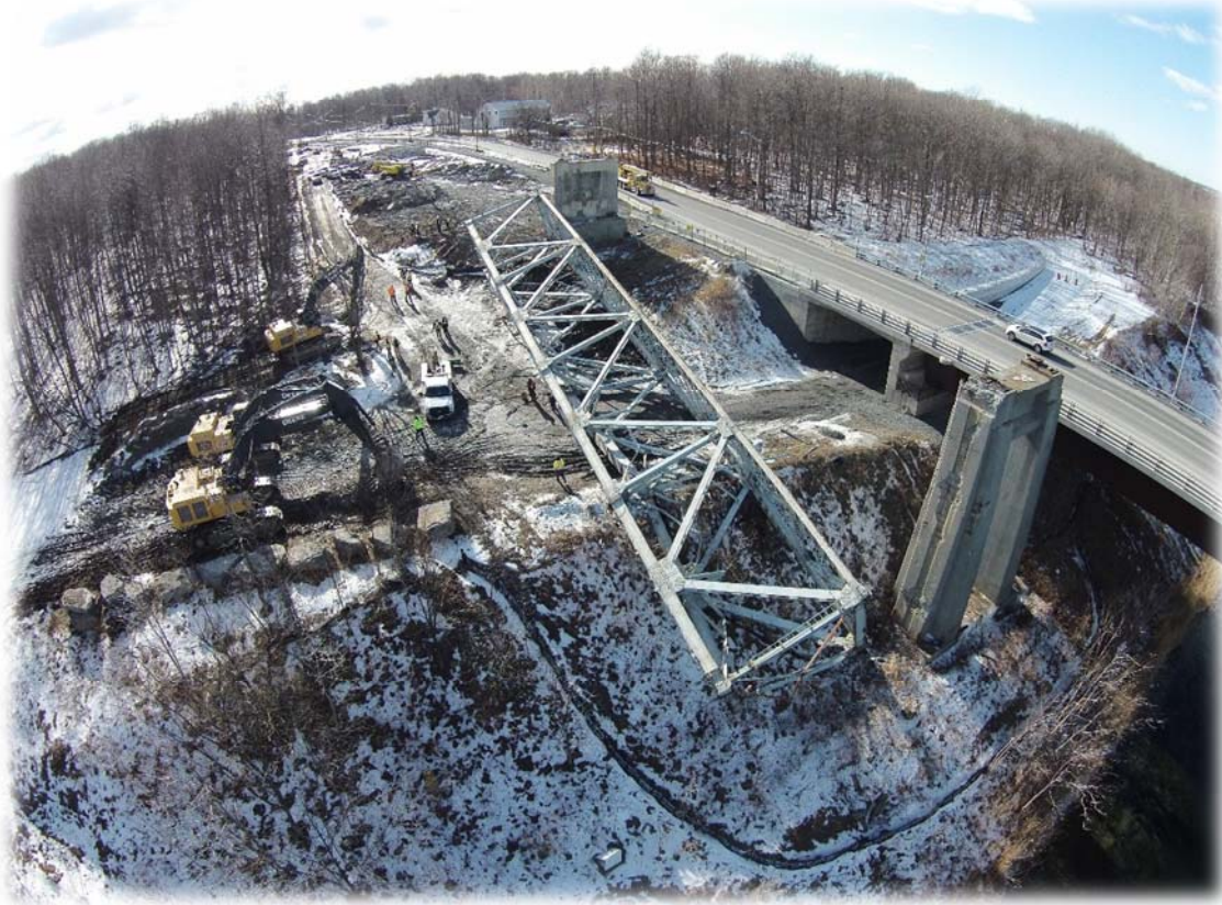
View of the dismantling of the very last steel structure on the old North Channel Bridge at the Seaway International Bridge in Cornwall.
