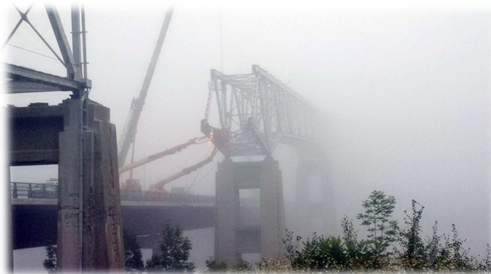
Dismantling the old North Channel Bridge at the Seaway International Bridge in Cornwall
