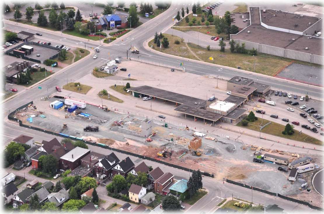
Aerial view of the Canadian Plaza work site in Sault Ste. Marie, Ontario
