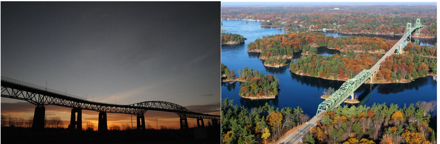
In Cornwall, the demolition of the old high-level North Channel Bridge will be initiated during Q2 (left). View of the Canadian Span of the Thousand Islands Bridge in Ivy Lea, Ontario (right). FBCL has also initiated the rehabilitation of the CBSA's Lansdowne Port of Entry project.
