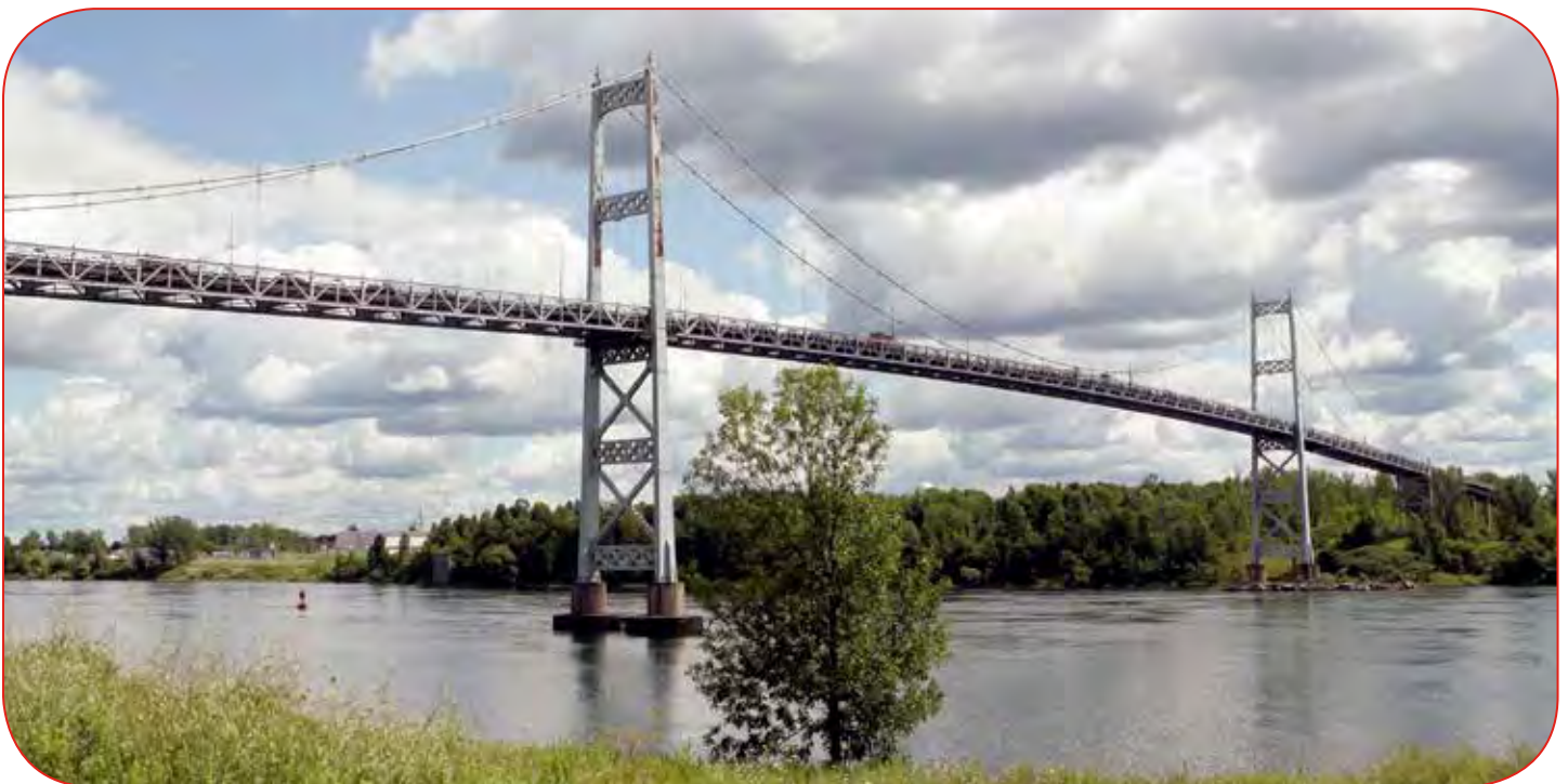
View of the South Channel Bridge between Cornwall Island and Massena, New York
