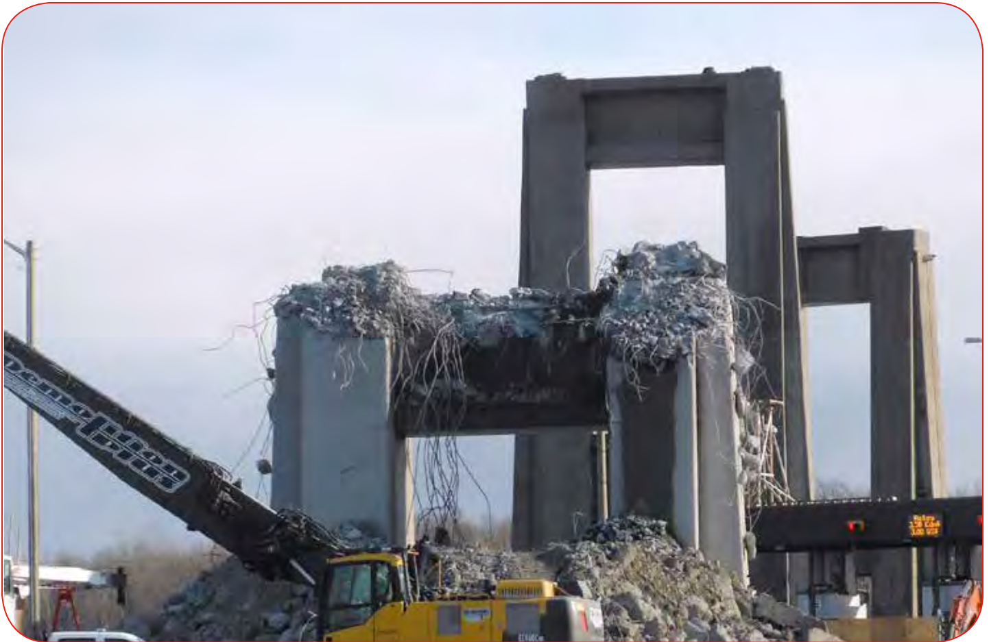
Toll collection in operation while the final phases of the North Channel Bridge demolition is underway at the Seaway International Bridge in Cornwall
