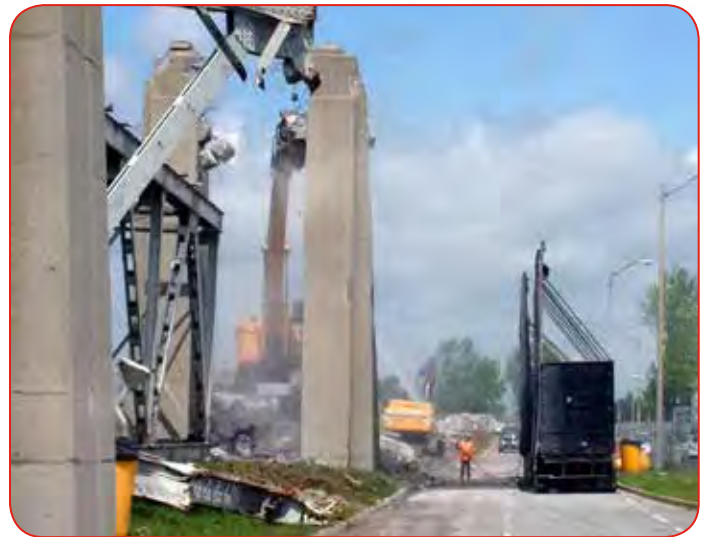
Pier demolition/steel structure removal in Cornwall
