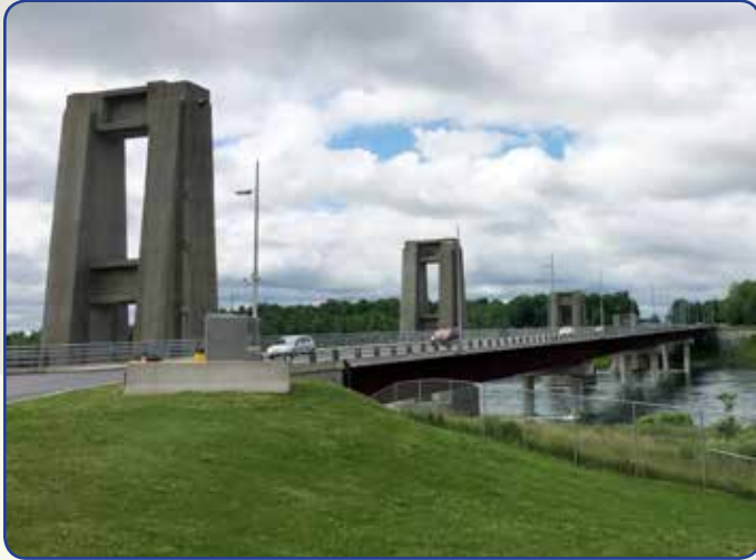
North Channel Bridge linking the City of Cornwall and Cornwall Island
