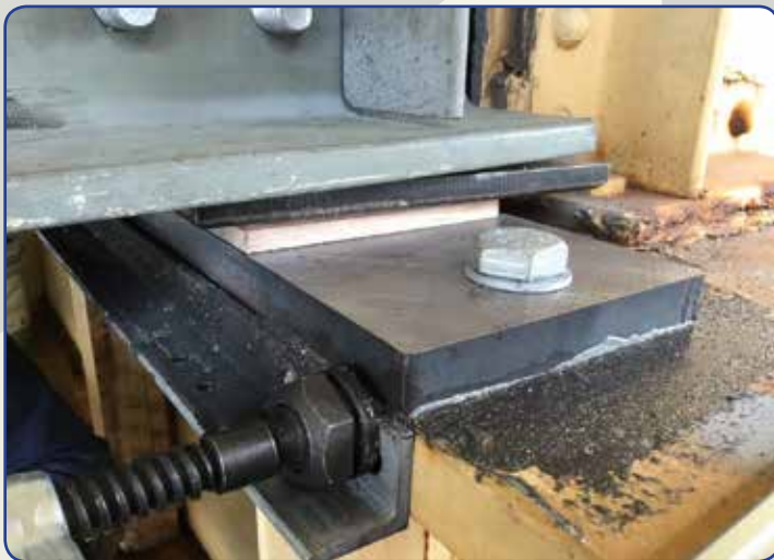
Steel bearing repairs at the Sault Ste. Marie International Bridge. The bridge is lifted with three 50 ton hydraulic jacks (photo courtesy of IBA)
