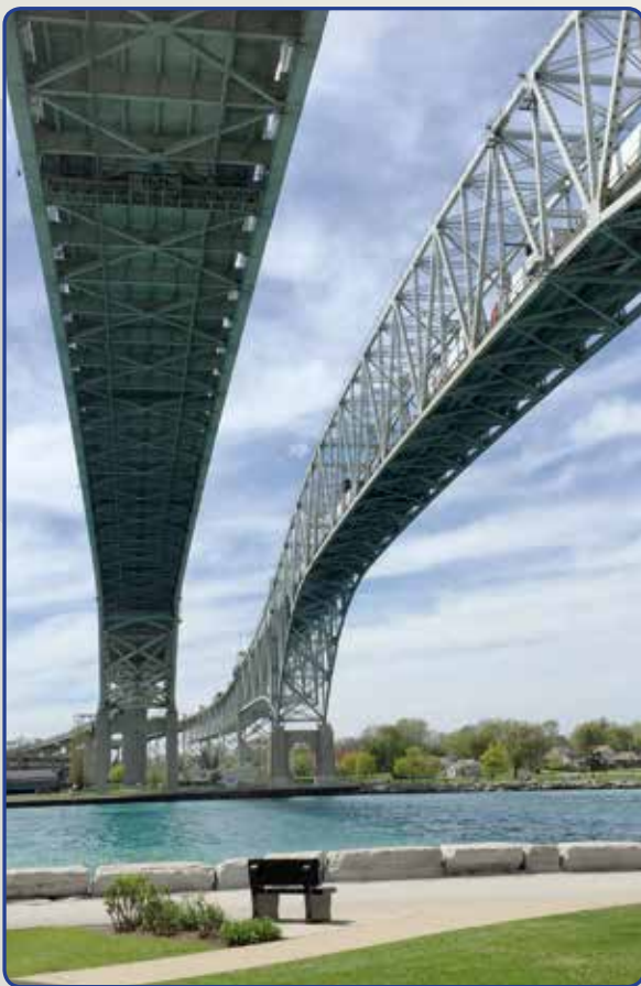
Blue Water Bridge in Point Edward, spanning the St. Clair River at the mouth of Lake Huron
