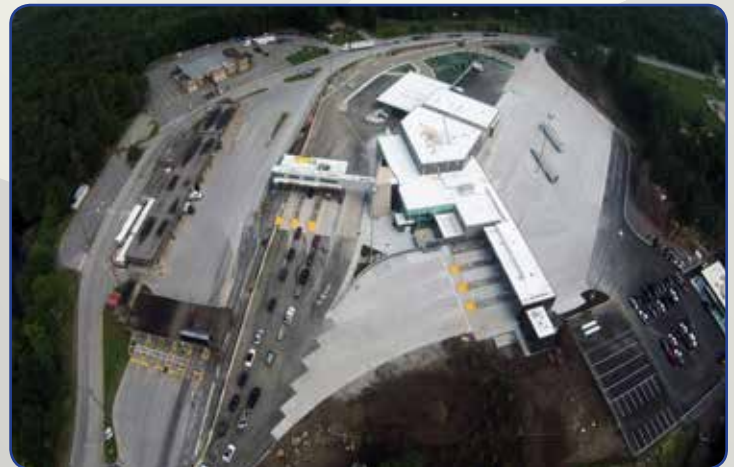
Aerial view of the new Lansdowne Port of Entry
