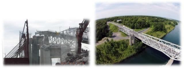
Ongoing dismantling the old North Channel Bridge at the Seaway International Bridge in Cornwall
